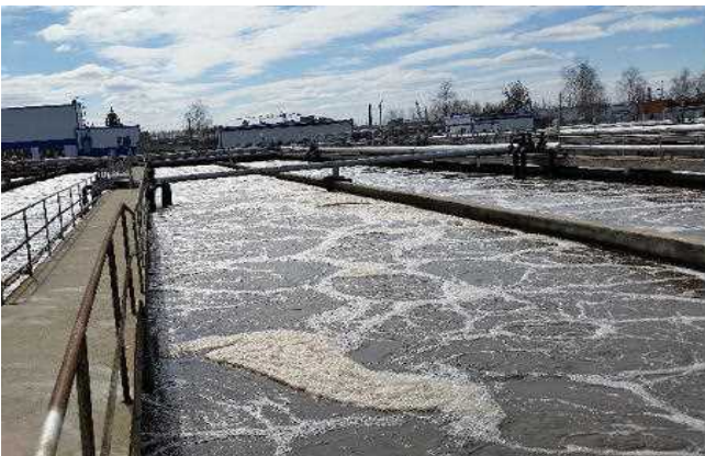
Fig. 12 Aging activated sludge tank (Russia)
