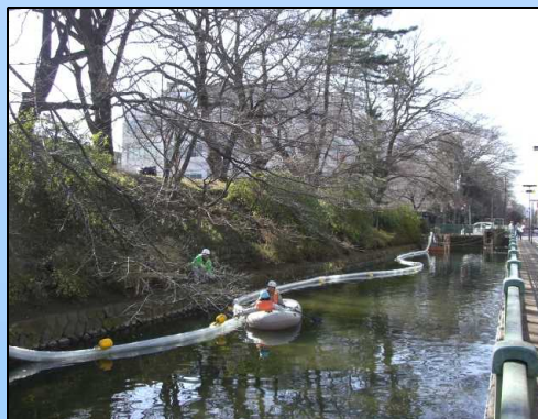
Mud water is sent to a treatment plant through pipes, to correspond to movement of the dredger, we set up pipes with floats on the water and set up laying metallic pipes on the ground.
