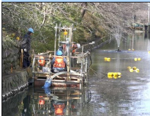
Sludge is mixed by an agitation pump on dredger. High concentration of mud water is sucked by a dredging pump.
