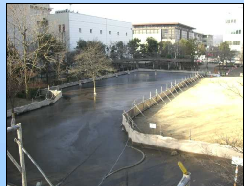
Muddy water which MSC agitated is released to a treatment yard and separates hydrophobicity immediately. There is no offensive odor during construction according to an odorless function of MSC.
